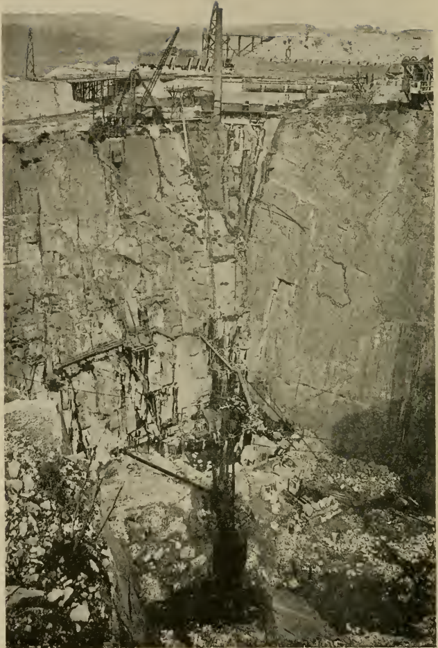
Granite Quarry, Kemnay
